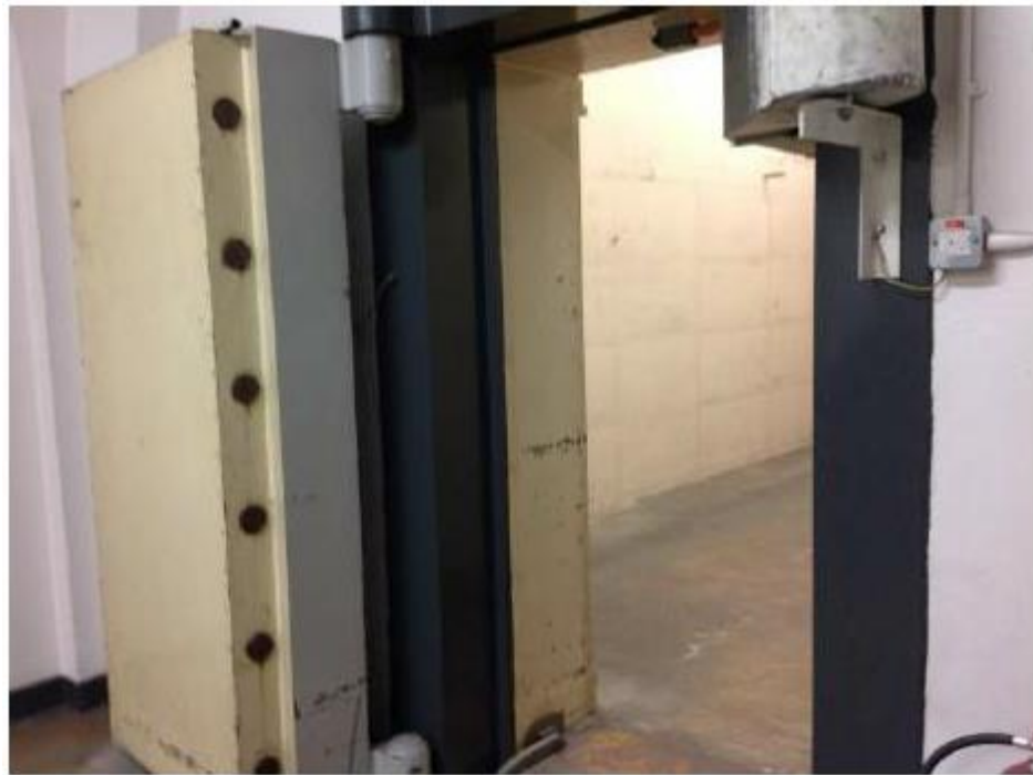
Images of Entrance Vestibule (top) and Basement Vault (bottom)
